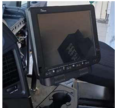
FM10Q VMC installed firmly on the truck
